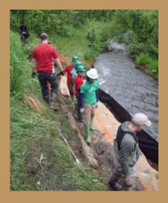
rehabilitate the area. At Ship Creek the crews placed straw logs to hold topsoil in place then a layer six to eight inches thick of topsoil. The crews filled in the area with 100 alder plantings and grasses.
