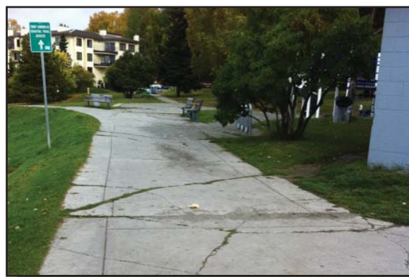
Pathways badly cracked and unsafe for bikers especially
