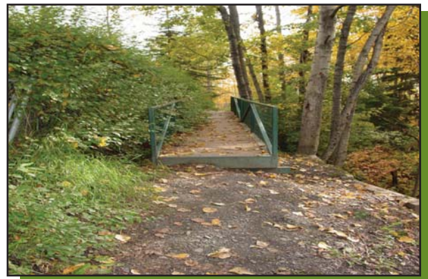
Users would like improved maintenance of the bridge and surrounding green areas
