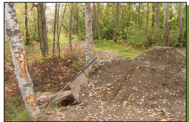
Erosion control work is needed in green areas
