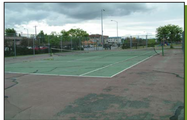
The tennis court needs nets and asphalt repairs
