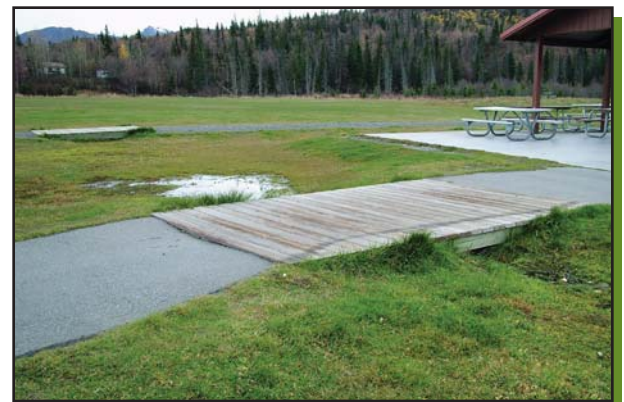
Poor drainage is a problem in this park
