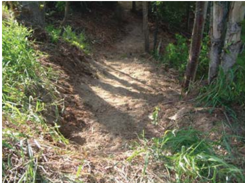
Before, a steep, eroding slope
