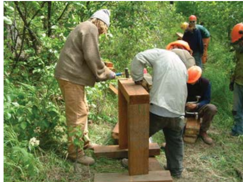
Community & Trail Crew Construction
