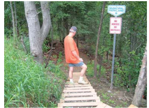
After! A sustainable & safe trail
