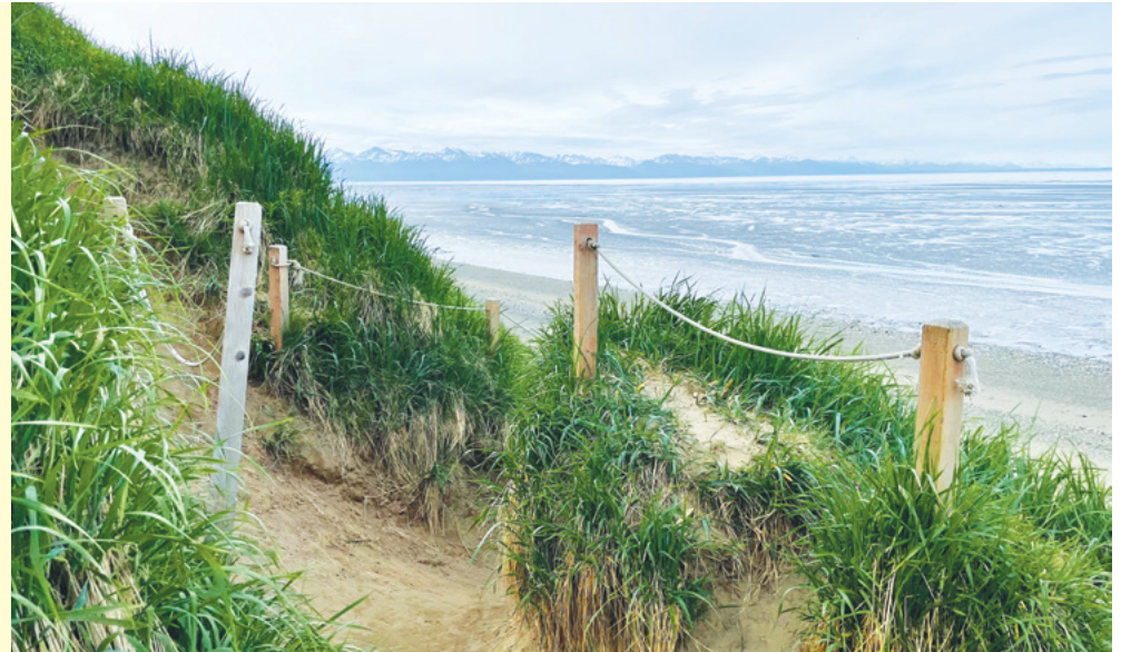
In 2015 Youth Employment in Parks built the 250 ft beach access trail. The teens also installed erosion control devices plus posts and ropes to minimize damage to dunes.
